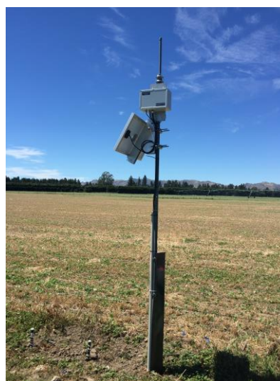
Pole mounted system
